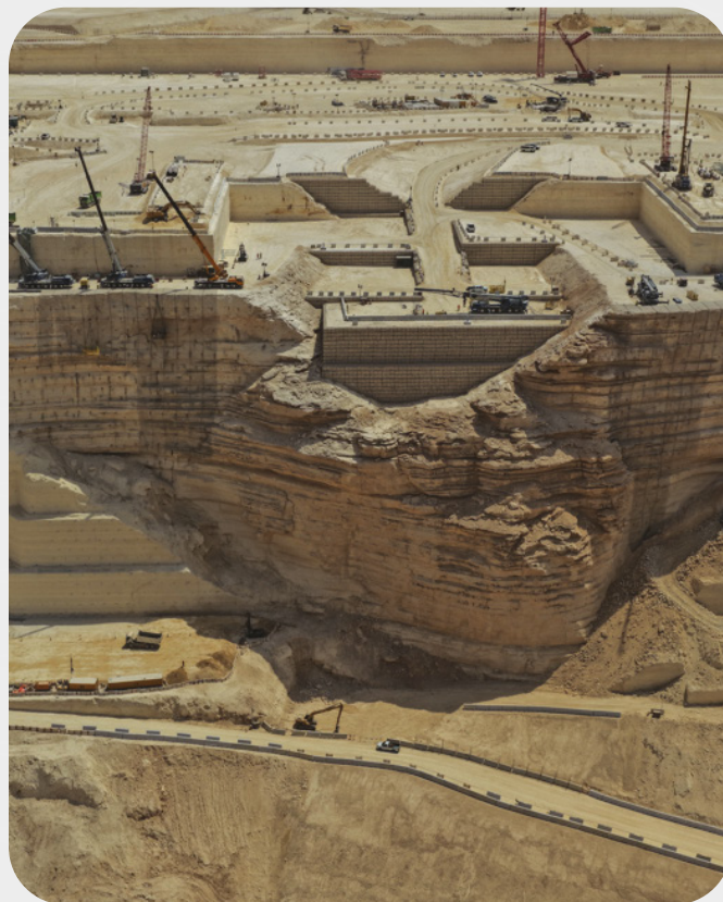
Credit @Populous: Build in progress for Prince Mohammed bin Salman Stadium, Qiddiya, KSA
